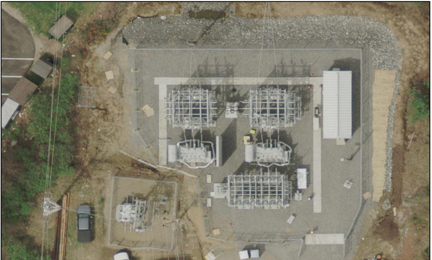
Aerial view of Substation #667 (South Sanford) located ~2.1 miles from the Site.
