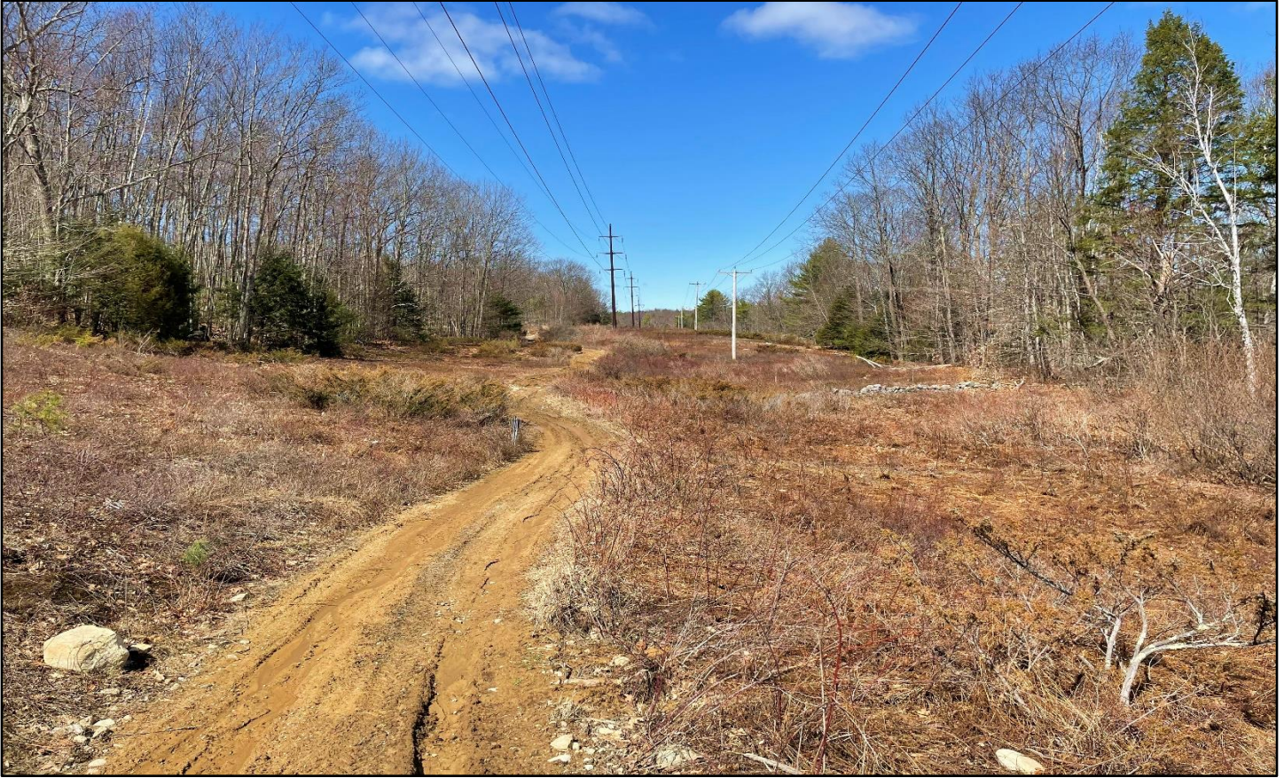
Photo of the transmission lines running through the Site.
